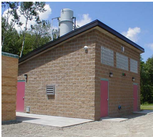
TCE Stripping Building
