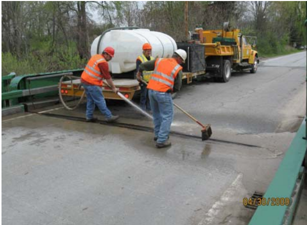
Members of the Allegany County DPW Bridge Maintenance Crew cleaning out a bridge joint
