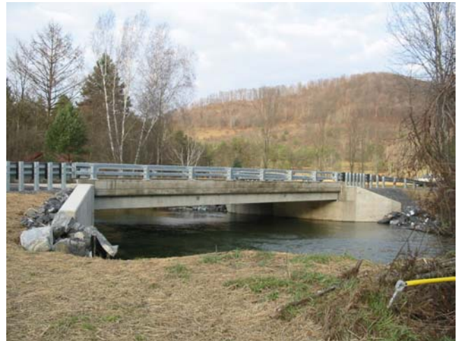
Fogel Crossing Road Bridge
