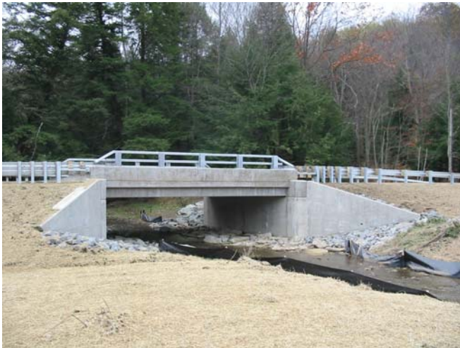
Champlin Hollow Road Bridge
