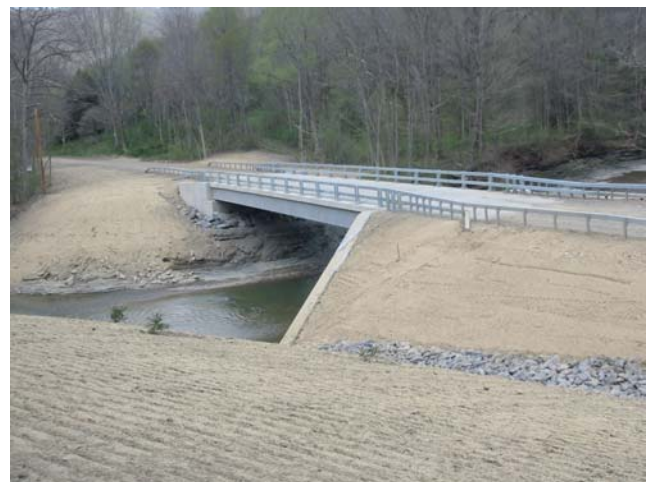
Figure 2: New Prestressed Box Beam Bridge
