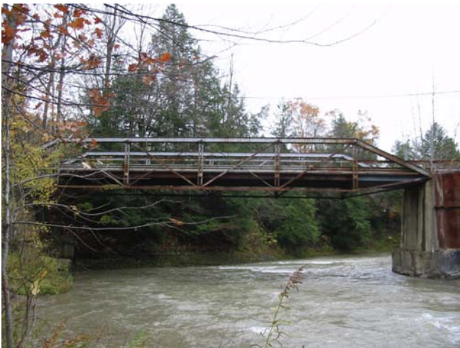
Figure 1: Former Pony Truss Bridge
